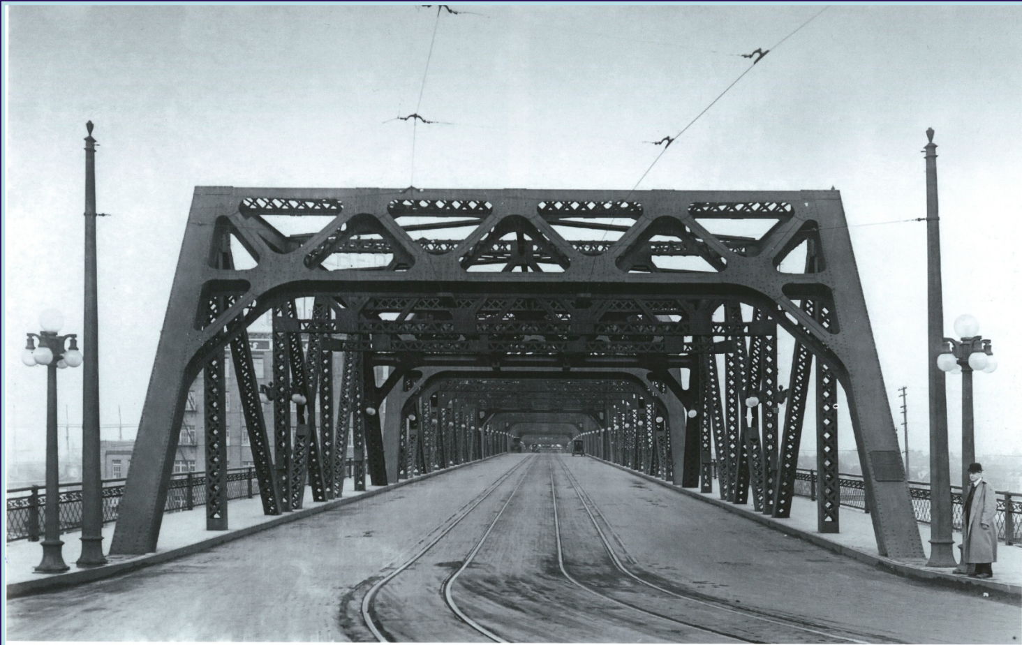
The Broadway Bridge opened in 1913 with streetcar tracks.
